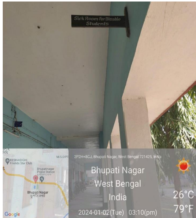
Figure 7: Dedicated rest room for disabled students
